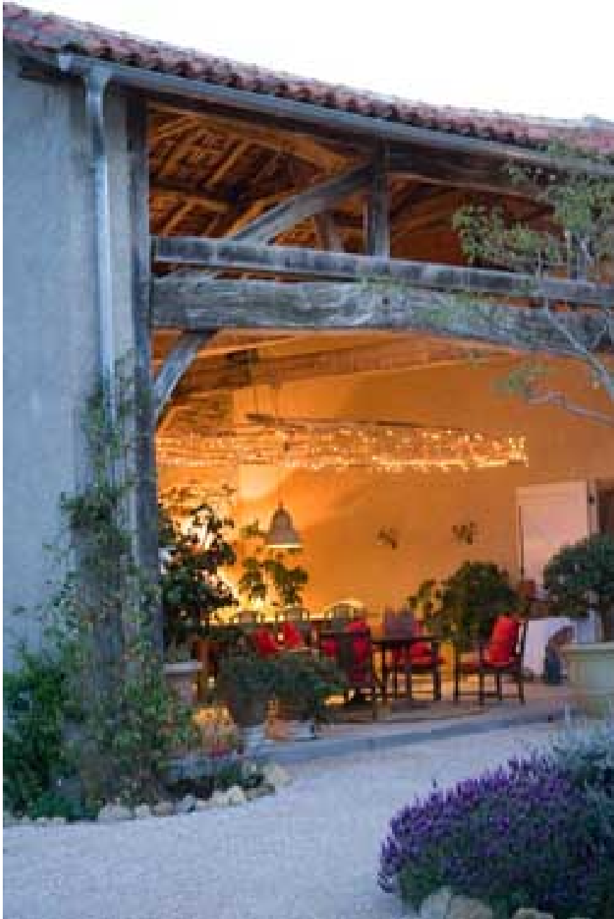
Tresbos Farmhouse France
