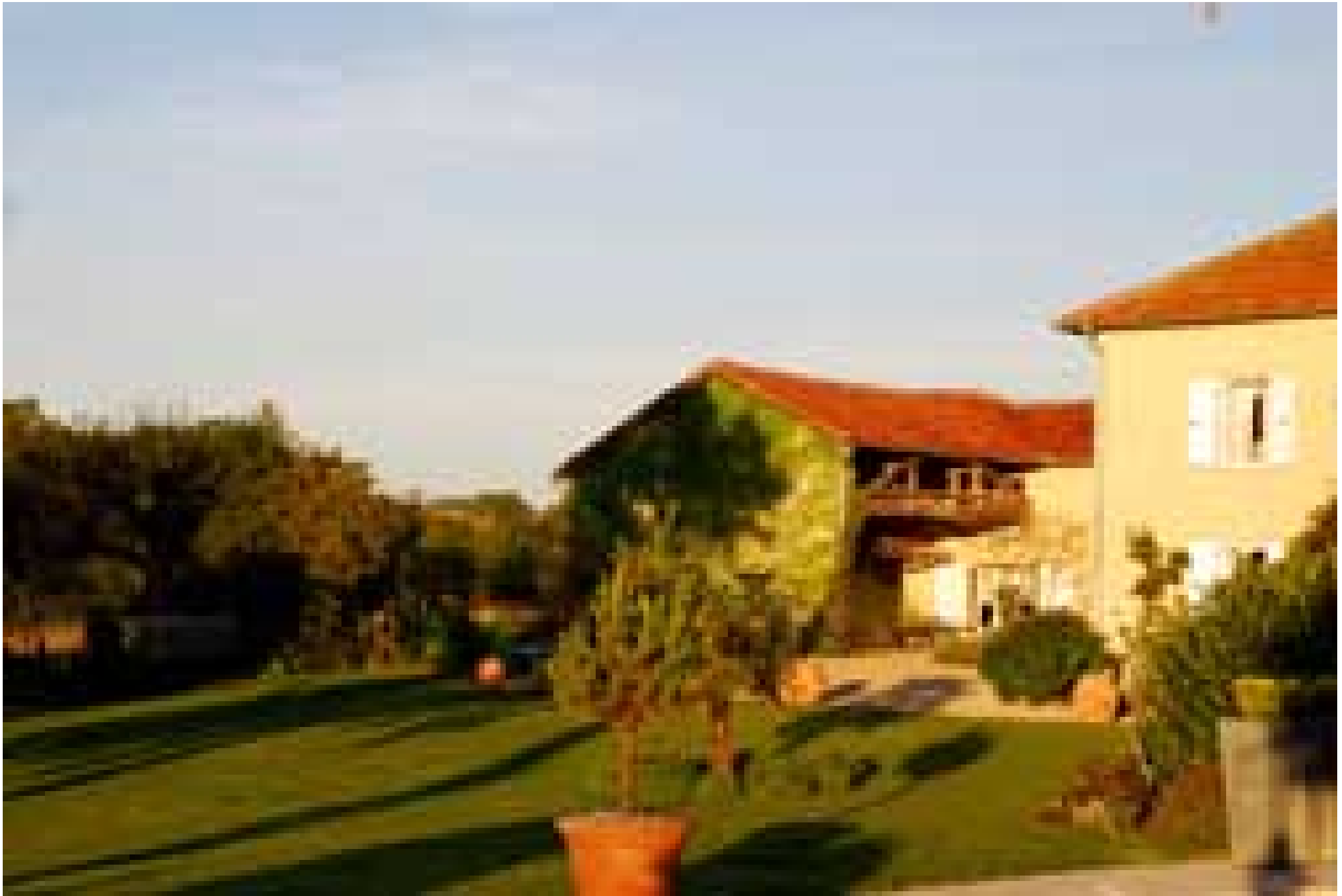
Tresbos Farmhouse France
