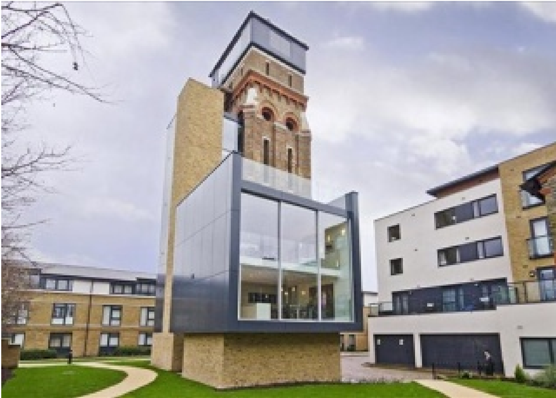
Water Tower SE11
