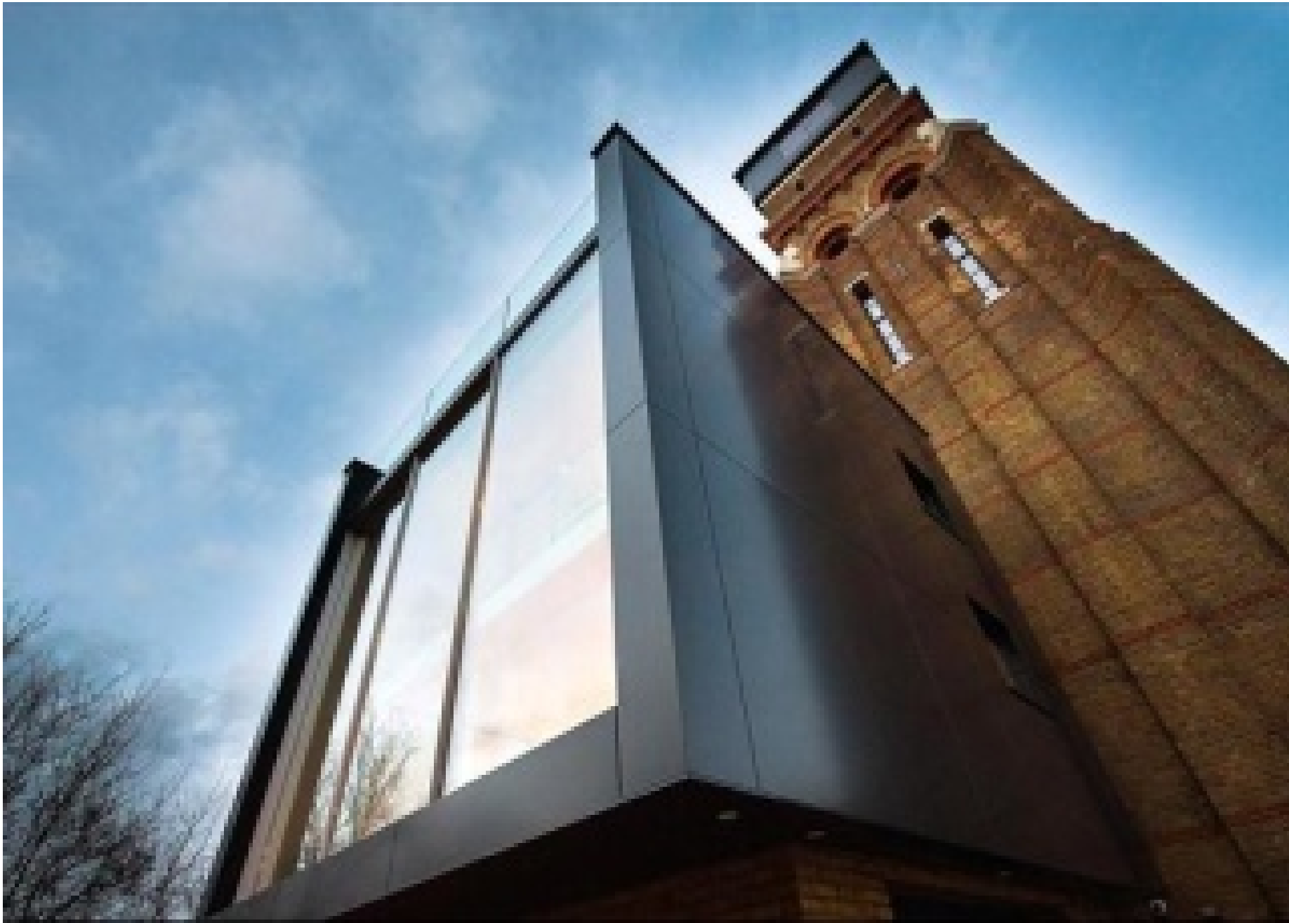
Water Tower SE11
