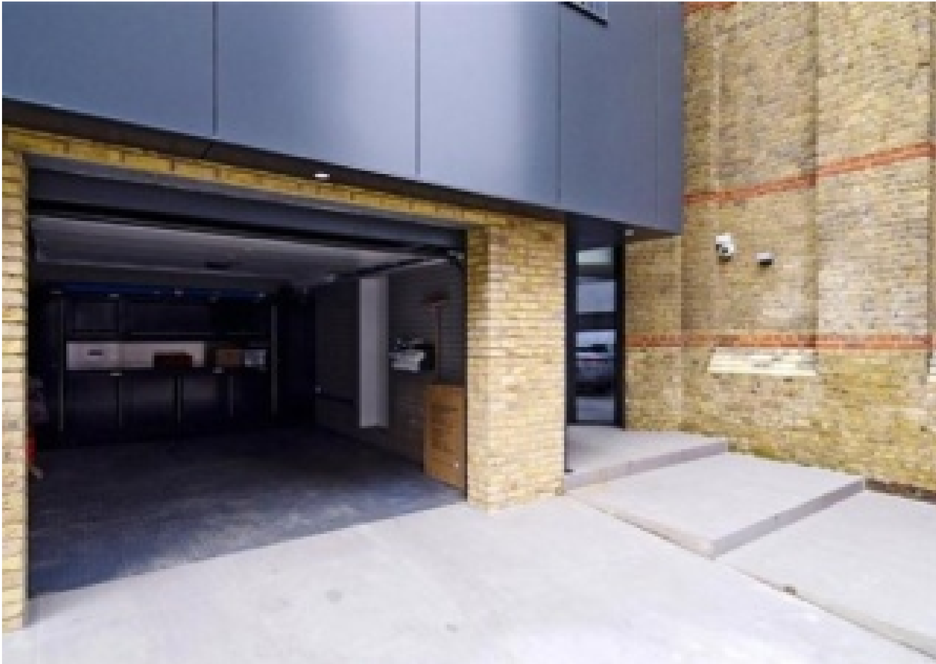
Water Tower SE11
